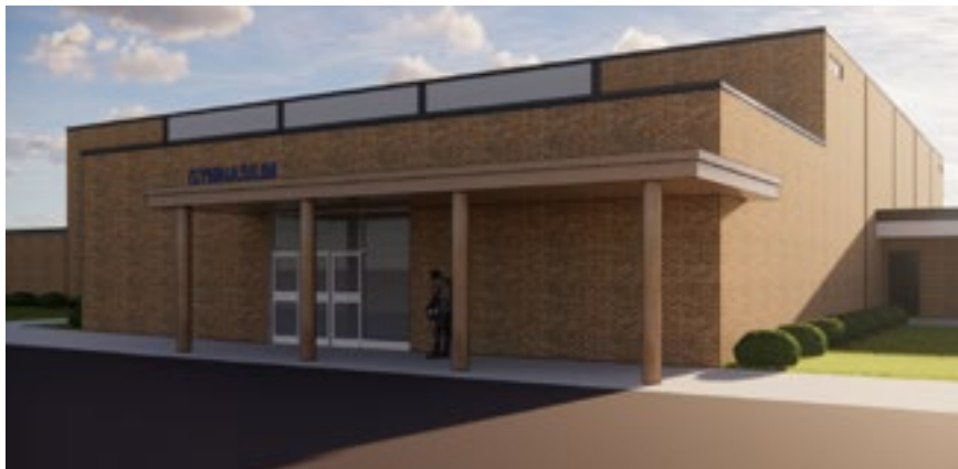
Addition to the high school gym
